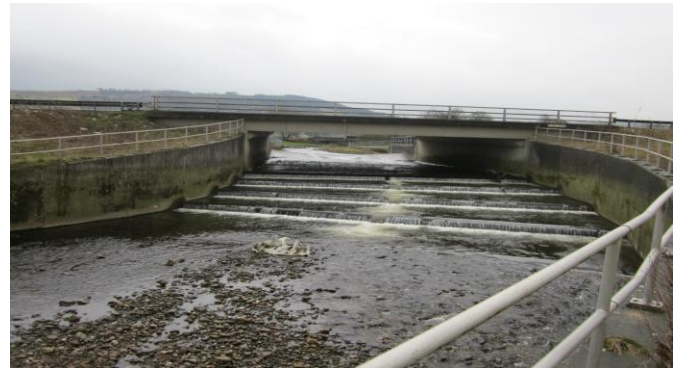
Looking upstream towards the bridge, lower weirs buried
